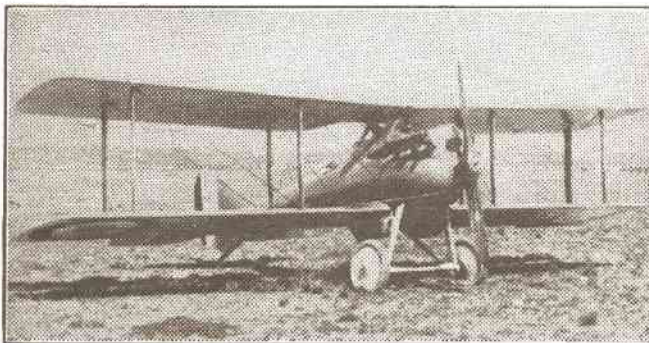
We understand that this 29C-1 was the last Nieuport made during the Big Fuss. She mounted the 300-h.p. Hisso. Note the twin Lambda radiators set under the wing roots. (Nieto photo).
