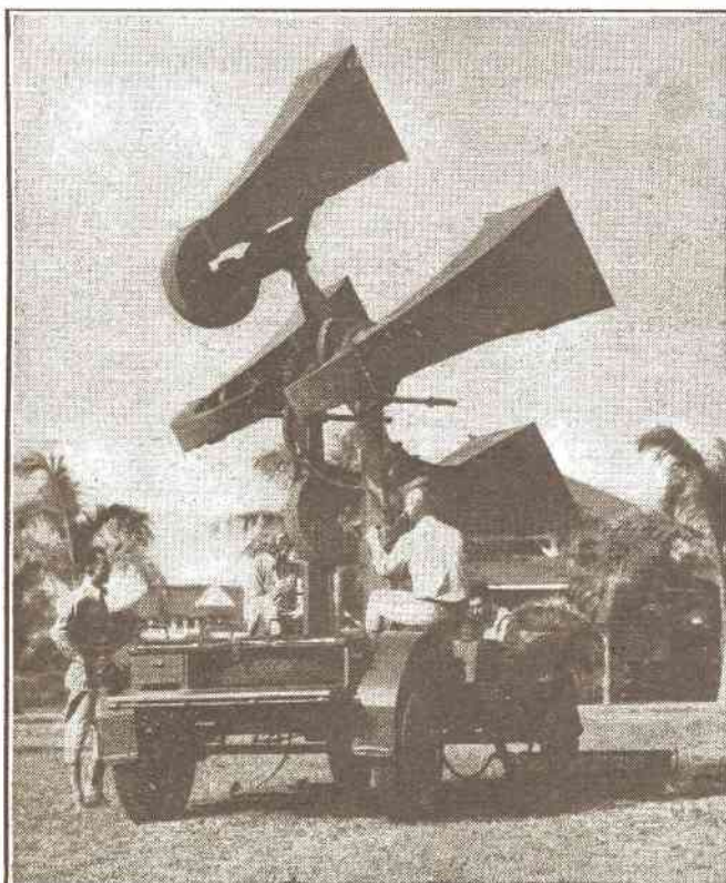
Invading air squadrons like to keep their approach a secret—but the secret's out once this sound locator is switched on! But the big question is: Have we got enough of these devices? The delicately-tuned horns catch the scarcely audible engine sounds of onrushing planes, and recording dials quickly indicate the direction of the attack. But the big question is: Have we got enough of these devices to comprise a real defence? (U.S. Signal Corps photo.)
